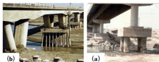
Fig. 1 Several types of complex bridge piers including pile groups, pile cap, and a column (a), some columns (b). (Yang et al., 2024)
