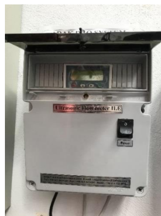
Fig. 4 Magnetic and ultrasonic flowmeters used in the laboratory
