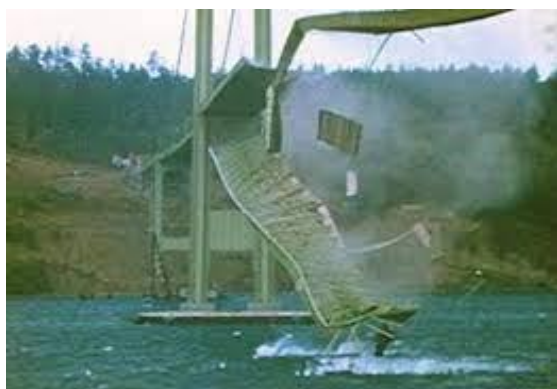
Fig. 2 Collapse of Tacoma Narrows Bridge due to oscillation and vortex shedding by the interaction of air fluid with structure
