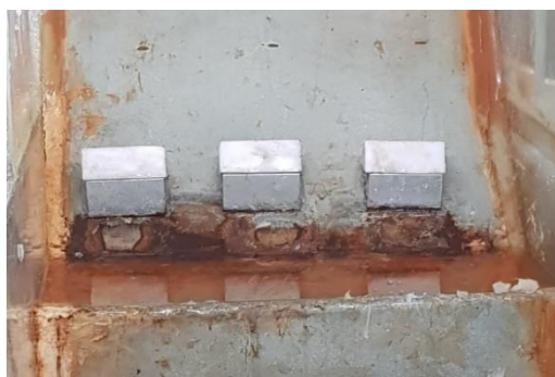
Fig. 4 A view of deflectors on flip bucket
