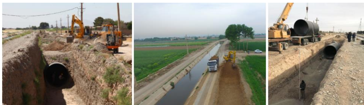
Fig. 16 Executive process of water conveyance line
