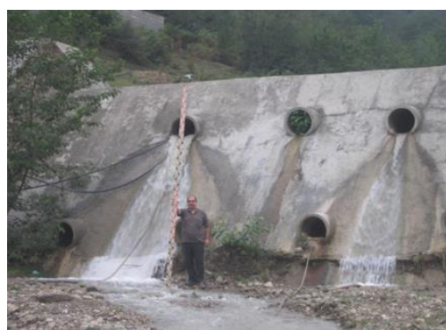
Fig. 3 Mapping downstream of Masonry check dam
